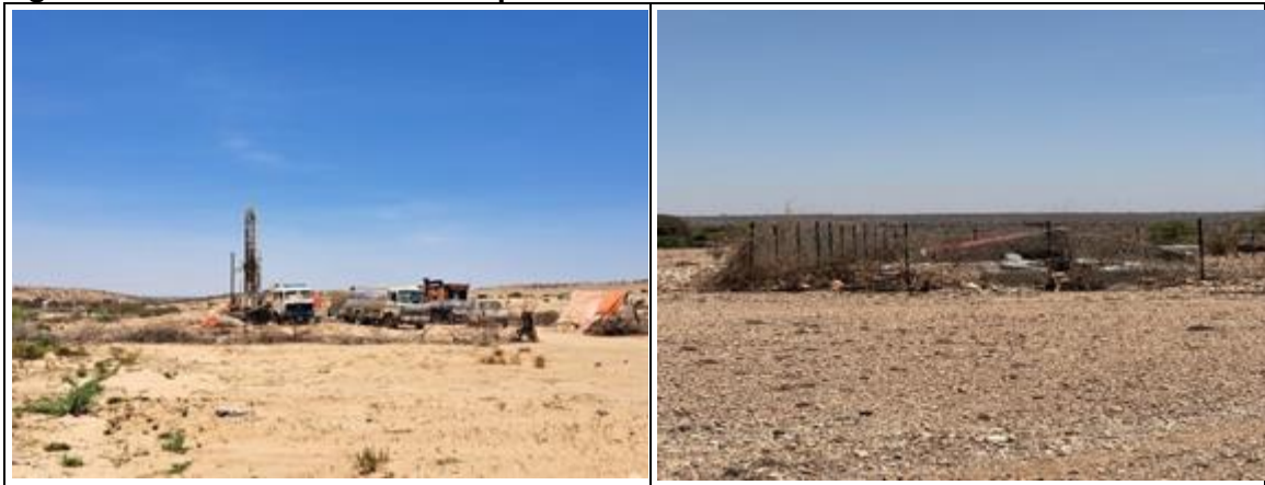
Figure 4-60: Borehole Under Development and Fenced Water Reservoir “Berked”.
