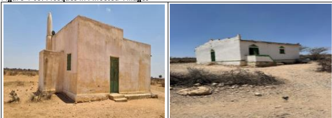
Figure 4-65: Mosques in Affected Villages
